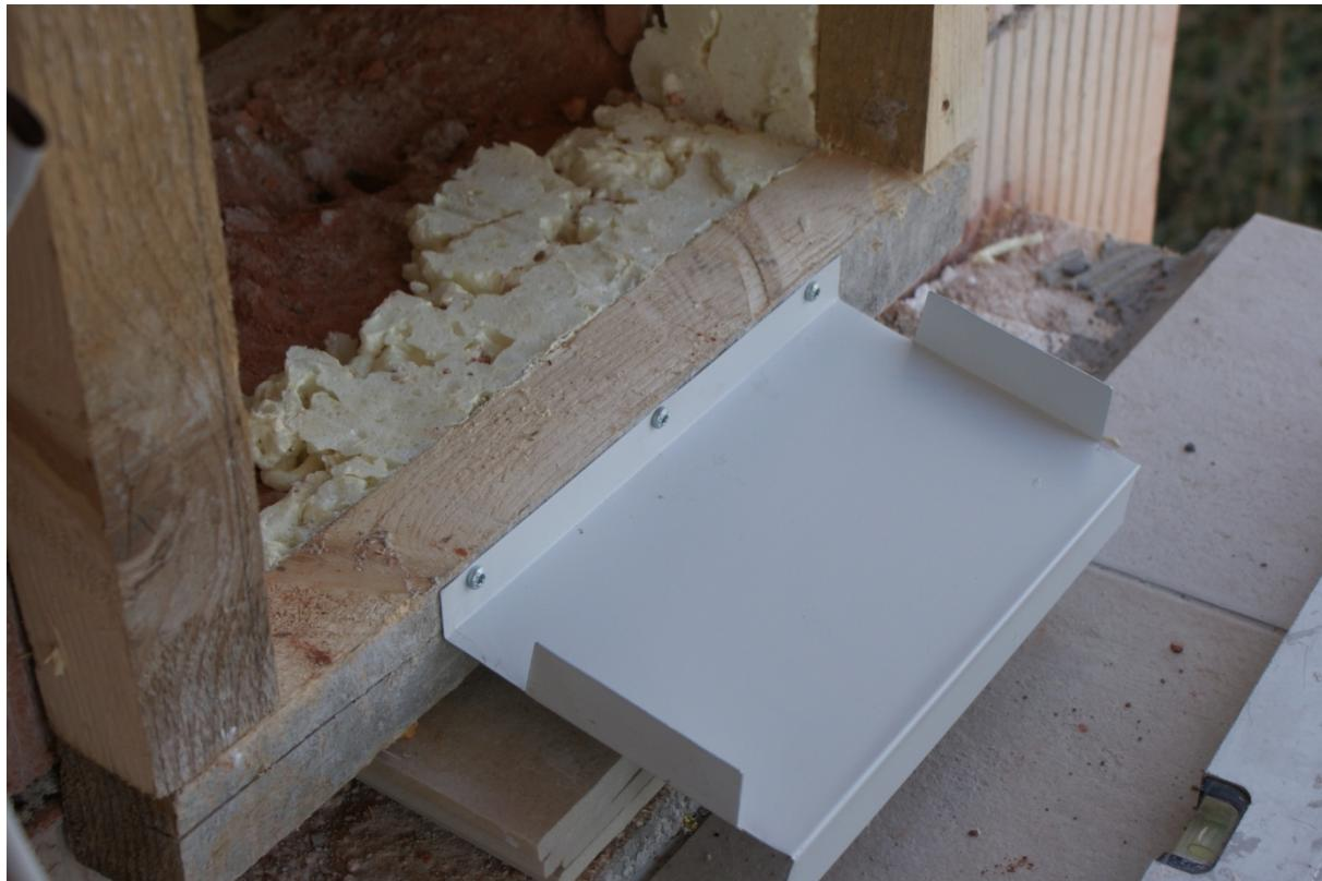
**Frame insulated mounting, i.e. the doorframe is covered by the thermal insulation of the building:**
